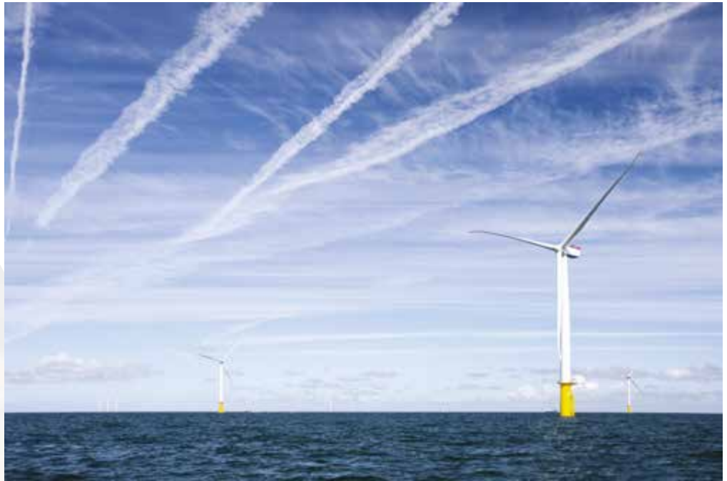
Hornsea Project One will produce enough electricity to power well over 1 million homes once it is operational in 2020. Photo courtesy of DONG Energy ©
