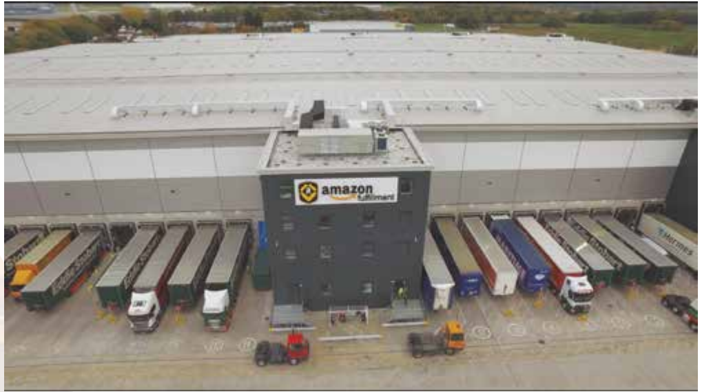
The new site at Airport City will be a pivotal distribution hub for Amazon, part of a growing logistical cluster in Manchester. Photo courtesy of Amazon ©
