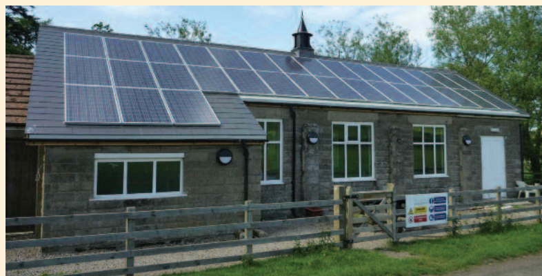
The heat pump will be powered, in part, by a 7kW solar PV installation
